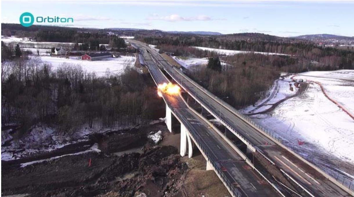
Drone-based bridge inspection and geodata provided by Orbiton after the collapse of Skjeggstad bridge on February 2nd helped determine that the bridge had to be demolished as quickly as possible due to danger of further collapse.
